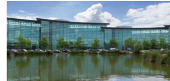
Reading International Business Park - Verizon UK HQ
